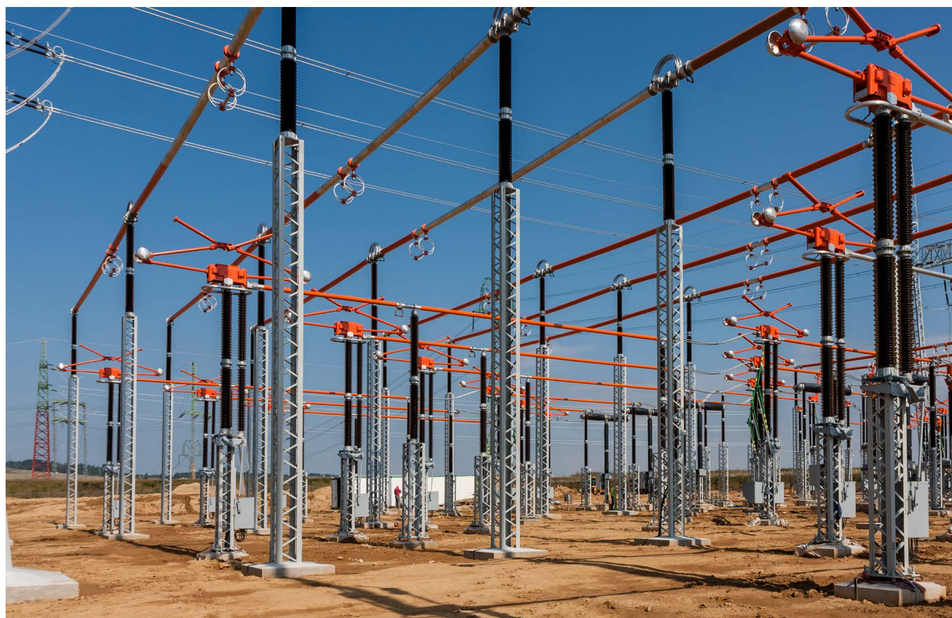
Pantograph disconnectors installed in a 420kV substation
