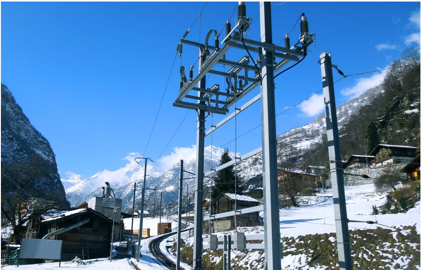
Railway - switch installed on portal
