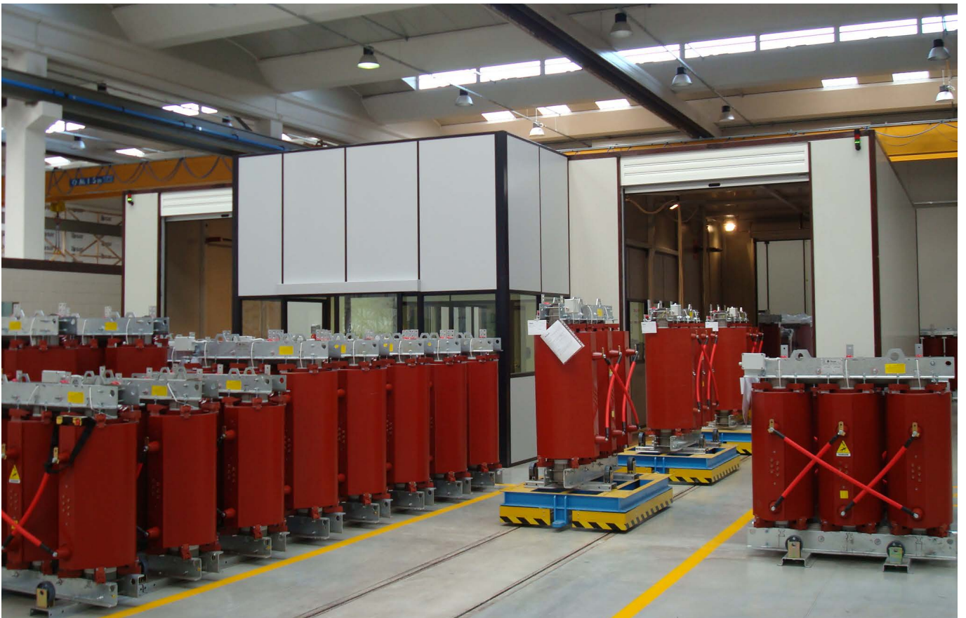
Testing bay for cast resin transformers
