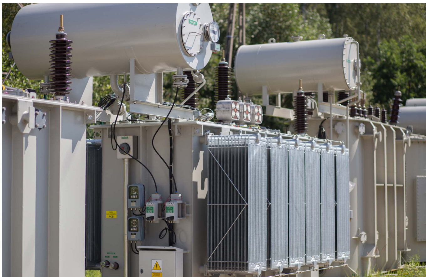
Power transformers waiting for transport
