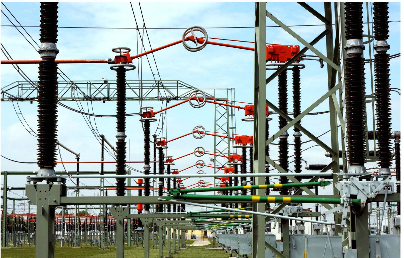
Vertical disconnectors 420kV with earthing switch
