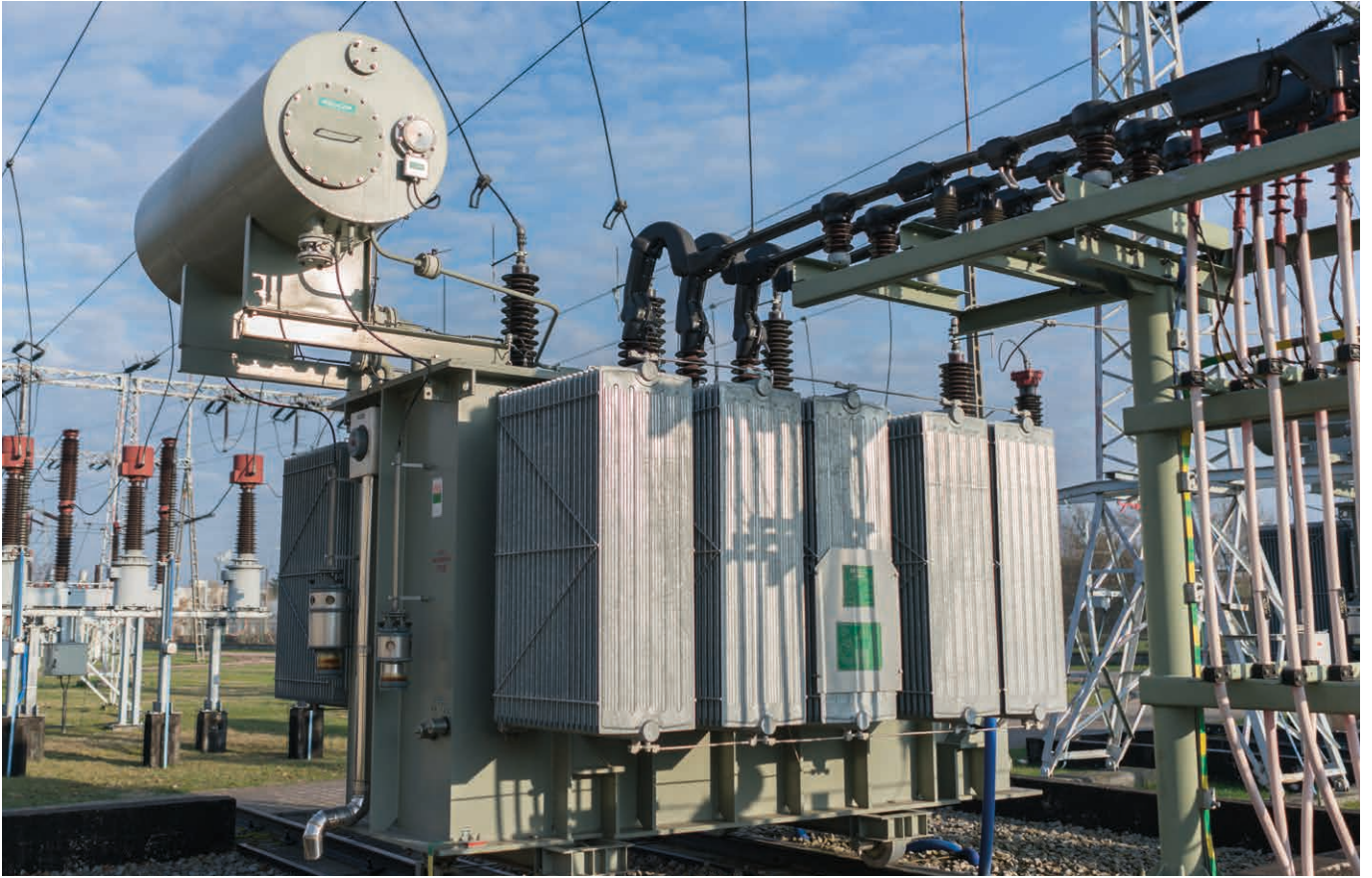
ZREW transformer installed in a substation
